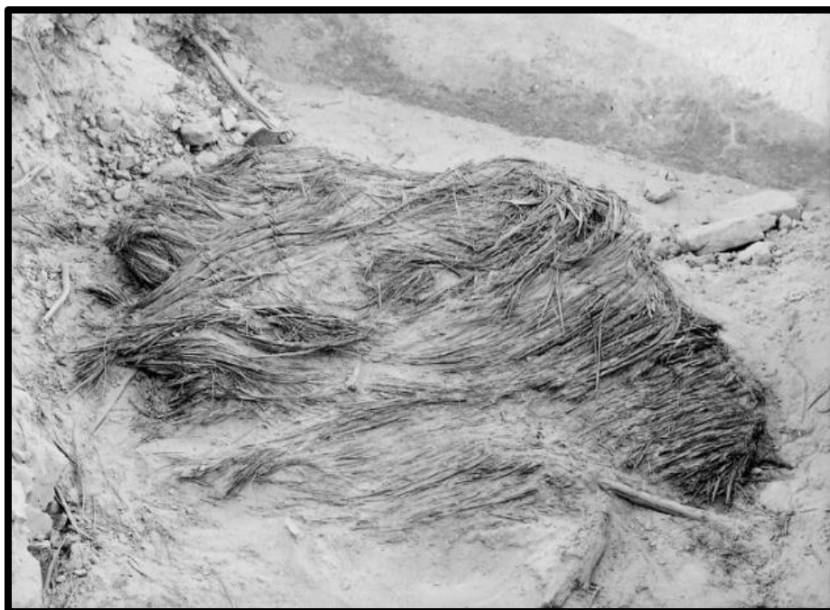
Figure 11: Remains of collapsed roof at #11 Gate Street
